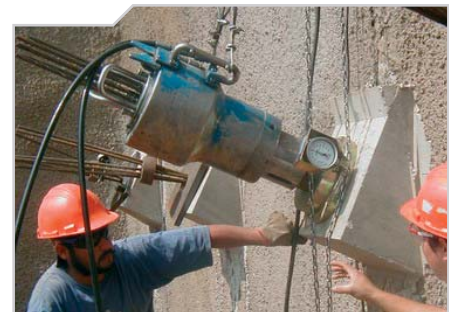
Stressing of anchor with load plate
