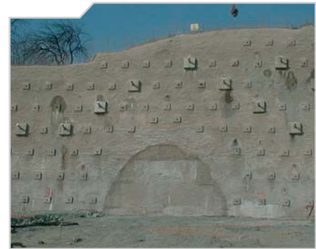
Portal support with load cells
