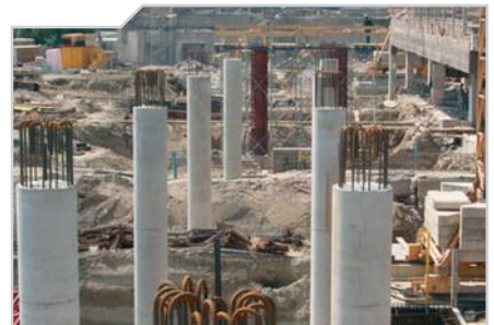
Little tolerances are permitted during bridge construction
