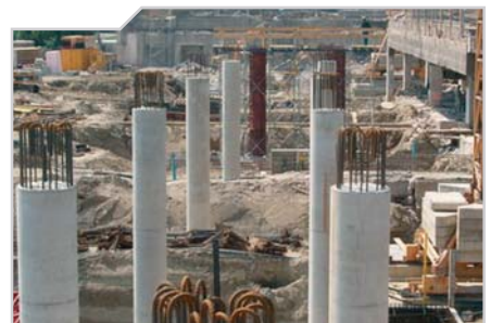
Little tolerances are permitted during bridge construction
