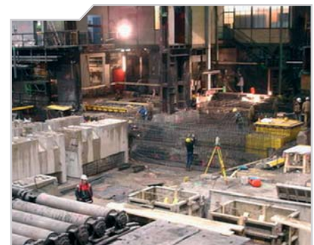
Setting out during reconstruction of a rail rolling mill
