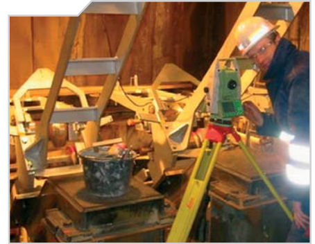
Setting out of in the bending area
