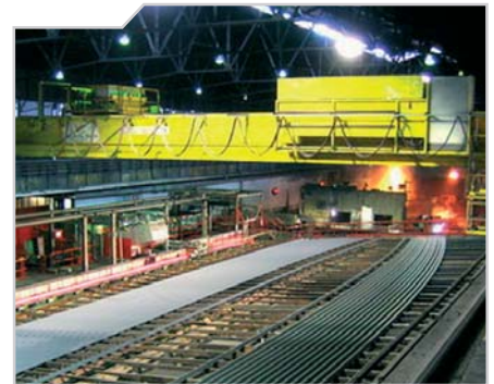
Surveying of the crane runway in rail roller mill
