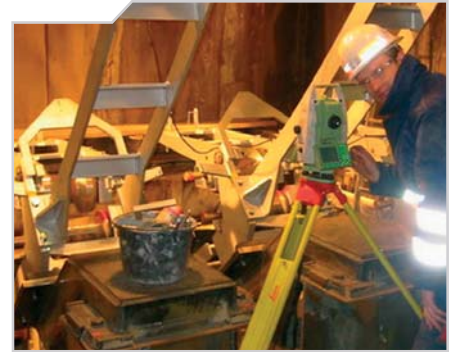
Setting out of in the bending area
