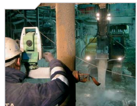
Setting out during reconstruction of a continuous casting plant
