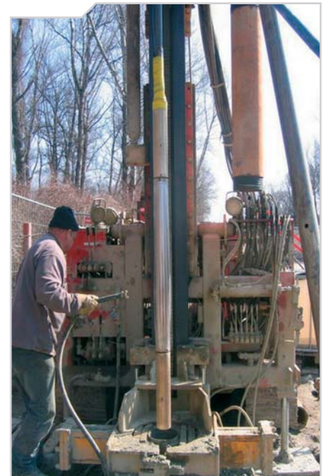
Installation of the dilatometer-probe
