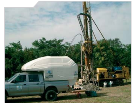
Dilatometer test for investigating the ground conditions for the future S1-free-way near Vienna
