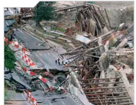
Tunnel collapse in Singapore
