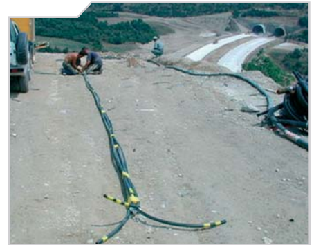
assembling of extensometers for a slope protection
