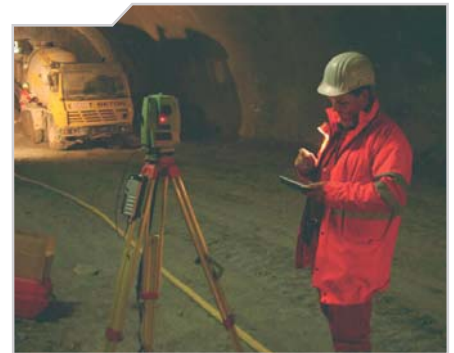
Controlling the final shotcrete layer with KRIOS
