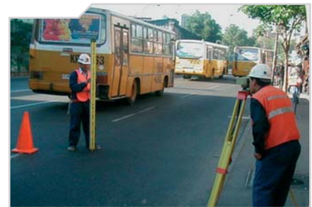
Precision-levelling during construction of Metro Santiago de Chile
