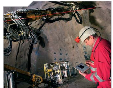
Setting out of drill holes by WLAN-Display
