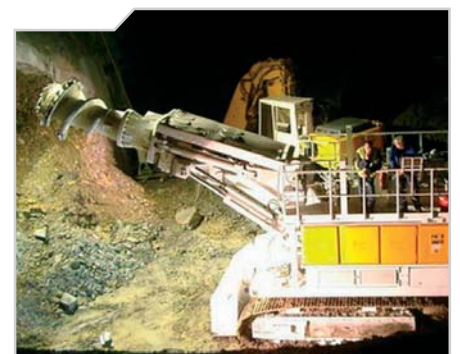
Roadheader with TAUROS guidance system during construction of the Achrain-tunnel, Austria
