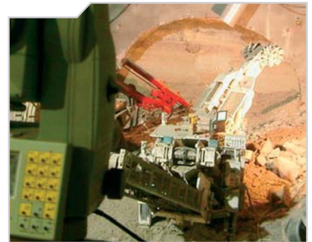
Steering of a roadheader at the CERN project
