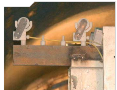
Covered targets on TBM
