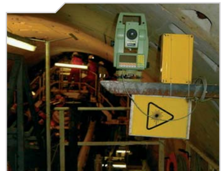
TBM guidance system on site
