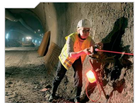
Continuous heading control with alignment laser...
